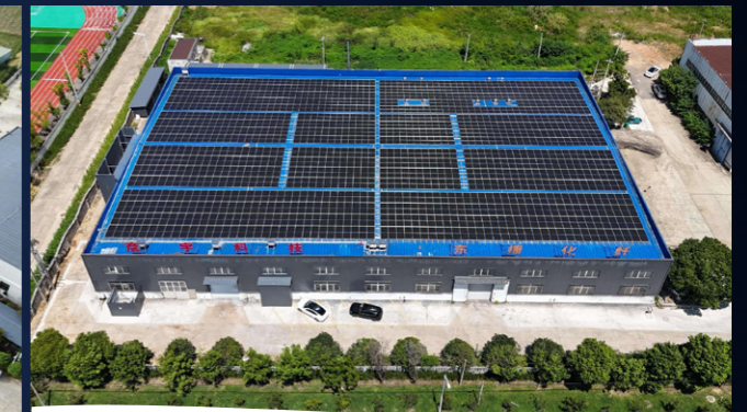
Warehouse, Italy 850 kW PV + 1.8 MWh BESS
