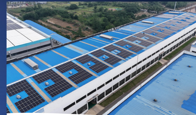
Factory, Indonesia 800 kW PV + 1.5 MWh BESS
