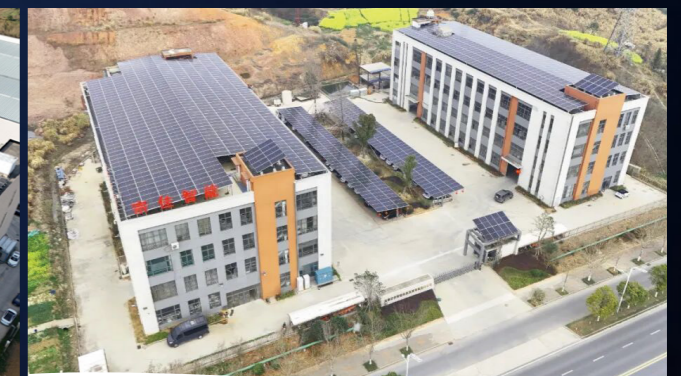
Factory, China 1.2 MW PV + 2 MWh BESS
